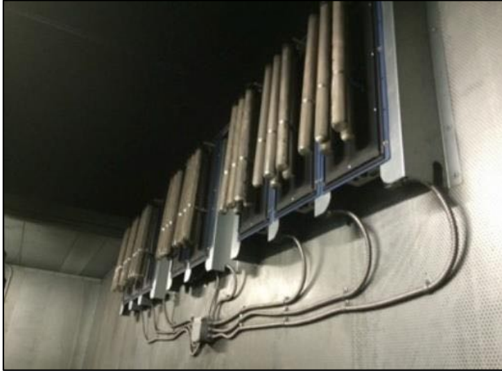
AtmosAir in Wall Mount Bracket (AHU/RTU)
