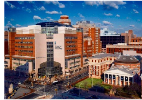
LBJ Hospital (TX) AtmosAir helped reduce VOCs by over 65%, and reduced five particle size ranges.
